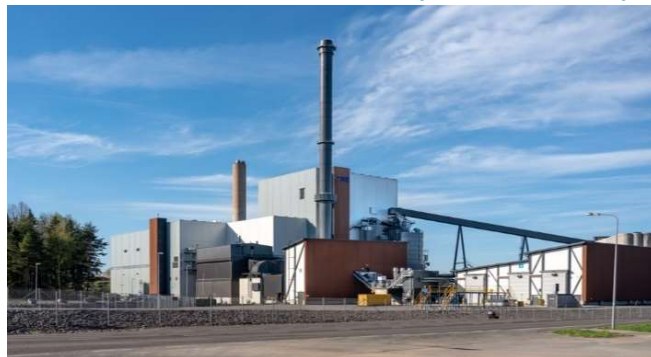
NA4 MULTI-FUEL COMBINED HEAT AND POWER PLAN, NAANTALI (430 MW), 18 100 m 2 , Completion 2017
