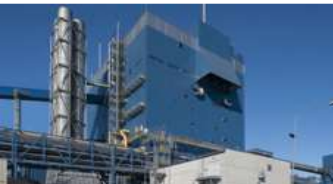
F3 EXTENSION OF THE FERROCHROME PLANT, TORNIO, structural engineering, 42 320 m 2 , Completion 2013
