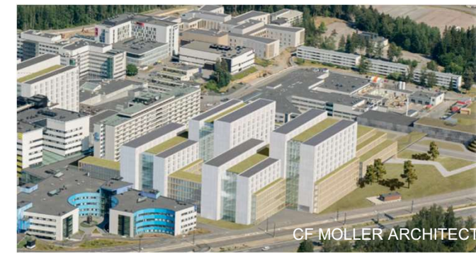
TAMPERE UNIVERSITY HOSPITAL, REFORMING PROGRAM 2030, TAMPERE, 180 000 m 2
