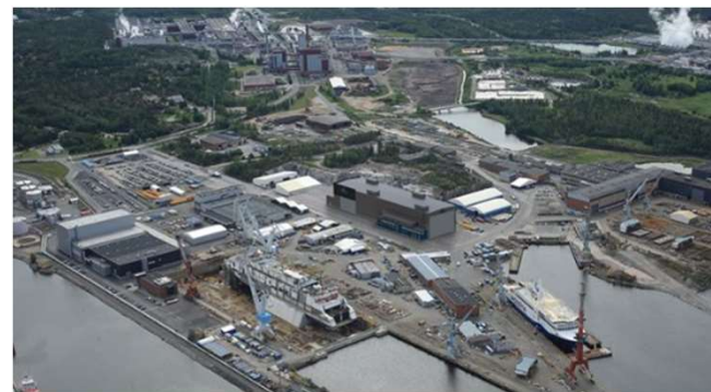
RMTK RAUMAN TELAKKA, SEASIDE INDUSTRY PARK, S-hallin laajennus 11 000 m 2 , Completion 2019
