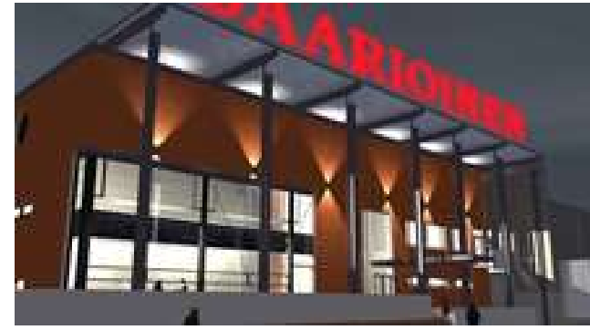
LOGISTICS BUILDING, SAARIOINEN OY 120 000 m 3
