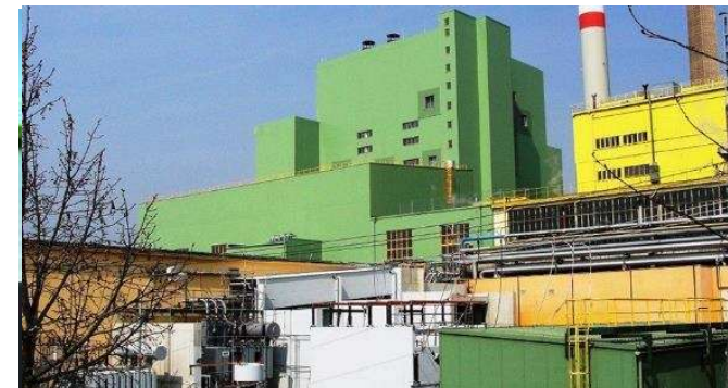
KLADNO POWER PLANT, CZECH, SUMITOMO SHI FW OY (135 Mwe, 303 MWth), Completion 2013
