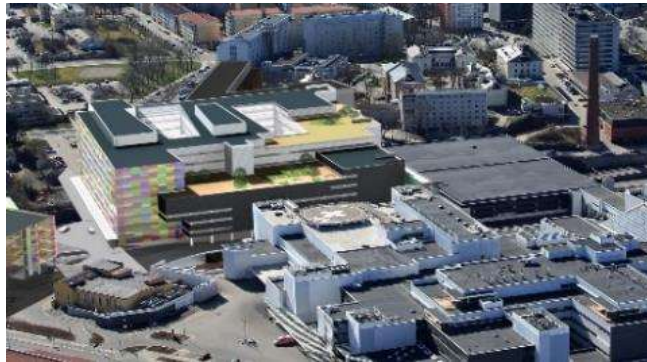
SOUTHWEST FINLAND HOSPITAL DISTRICT, "LIGHTHOUSE", TURKU, 53 600 m 2 , Completion 2021
